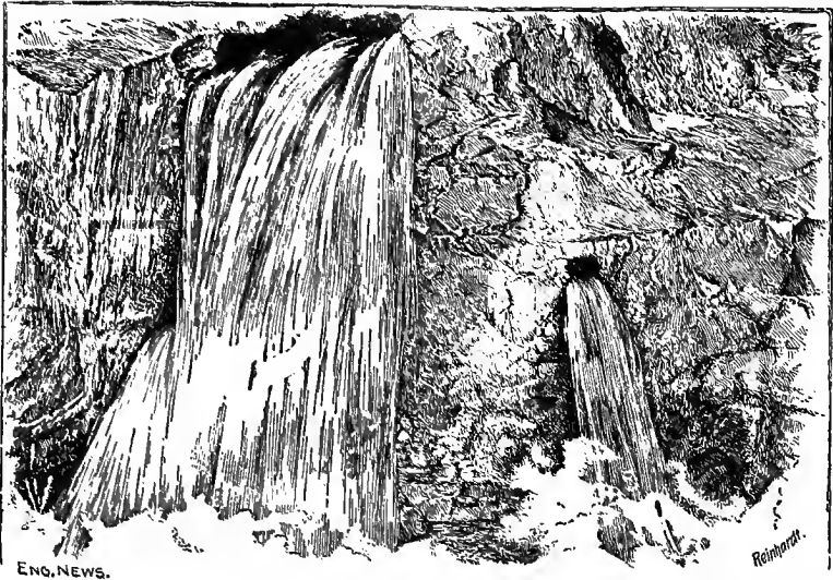
FIG. 122. — Sketch Showing Underground Stream, Milwaukee Water-Works Tunnel.
